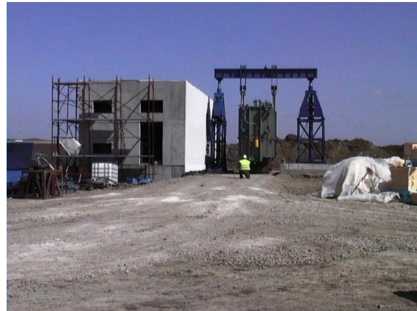
Installation of the transformer in the foundation
