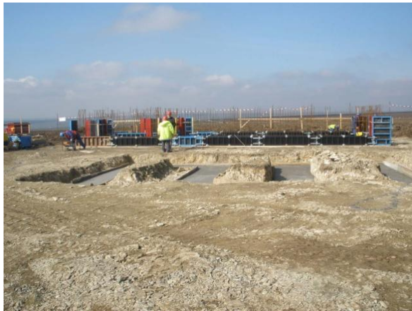
Foundation of FE substation
