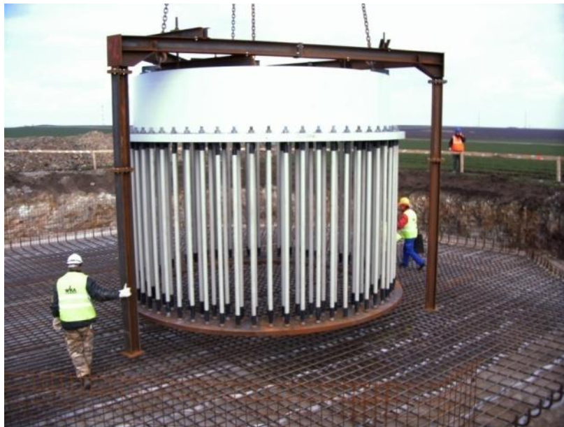
Placing of adaptor to foundation
