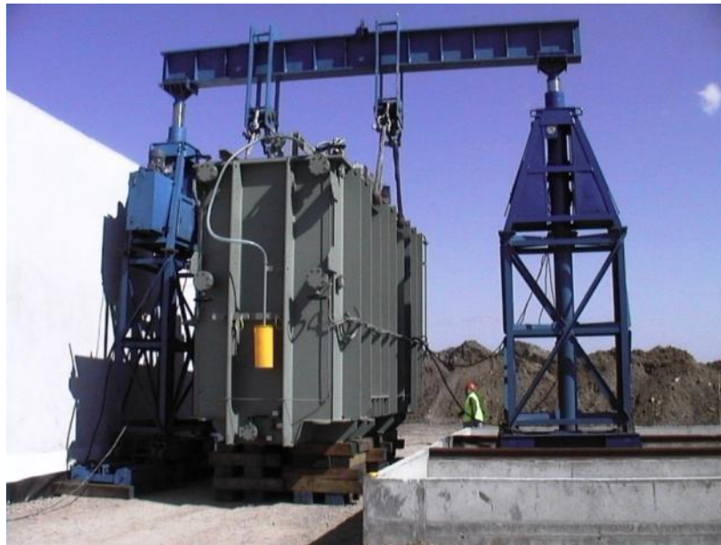
Delivery of the 1 st transformer for FE substation on site
