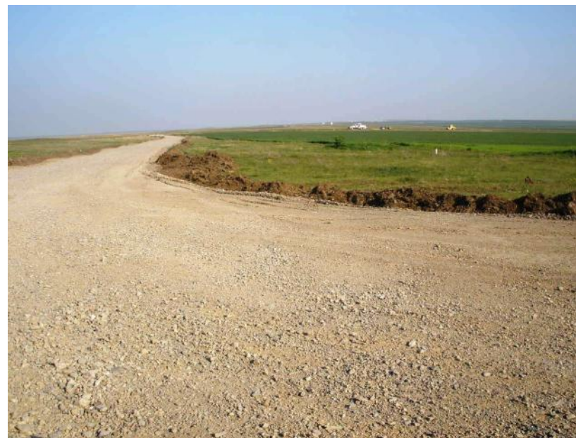
Start of the works for MTS roads
