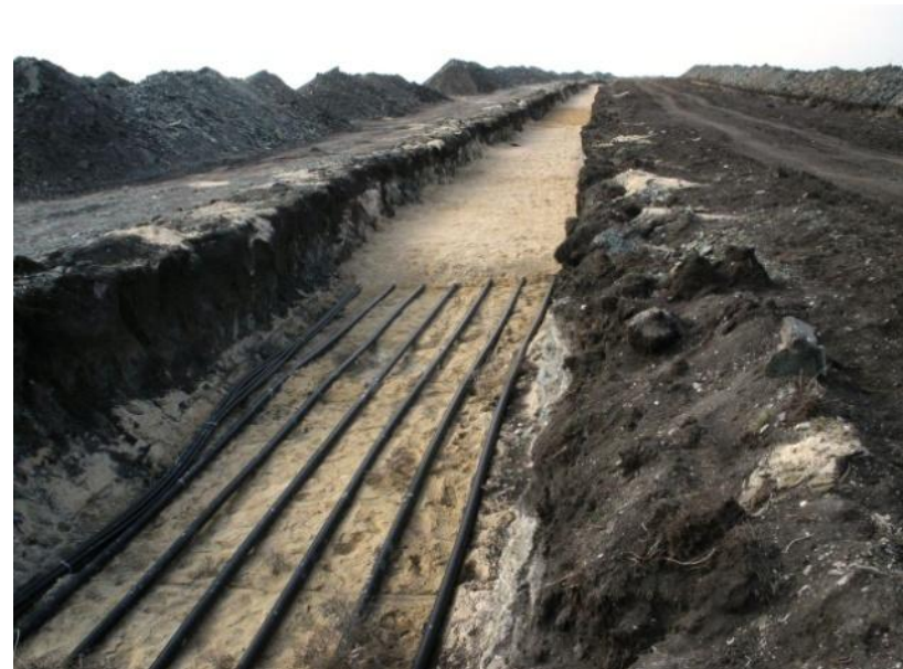
Laying of 110 kV cables
