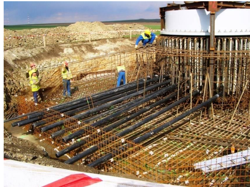
Placing of cable ducts into foundation
