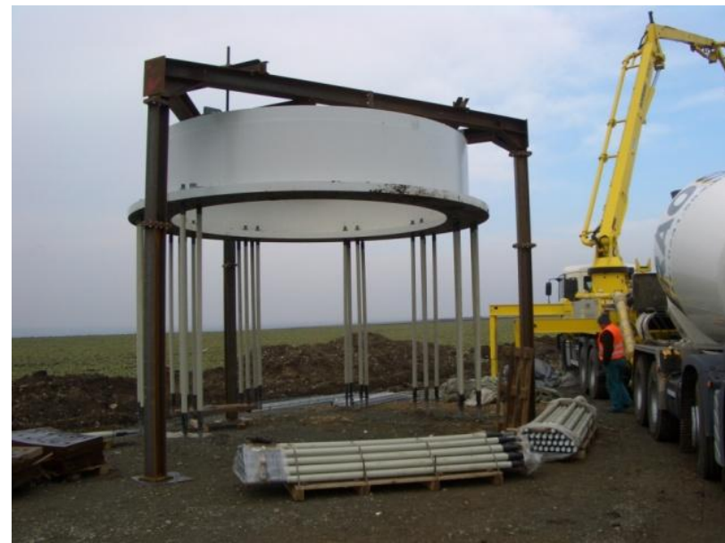
Construction of adapter ring and steel installation
