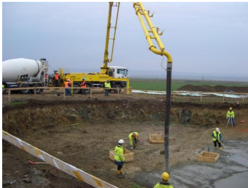
Pouring of blinding concrete
