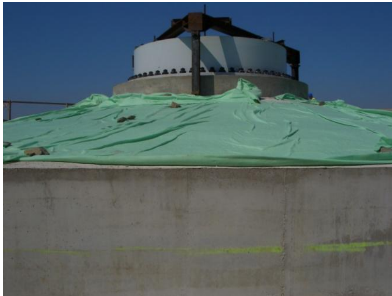
Finalization of concrete foundation FE17
